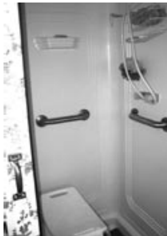
Grab bars added to shower enhance safety and comfort while bathing.
